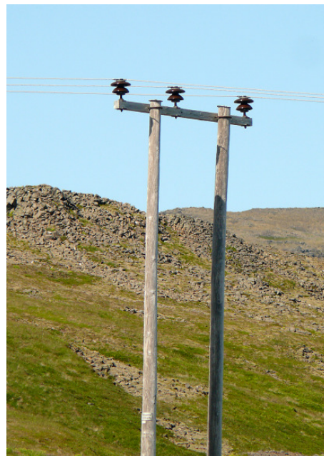
Figure 4. Left: a safe horizontal low voltage line, with three conductors suspended below cross-arm with sufficiently long insulators. Right: a low voltage line in Iceland unsafe for larger waders, here Whimbrel ( Numenius phaeopus ) and Black-tailed Godwit ( Limosa limosa islandica ) and larger raptors (in this case White-tailed Eagle ( Haliaeetus albicilla ) and Gyr Falcon ( Falco rusticolus )) because of conductors attached on short insulators on top of cross-arm. In this case retrofitting could include insulating the central conductor wire and/or covering the insulators (Photo: Bureau Waardenburg).
