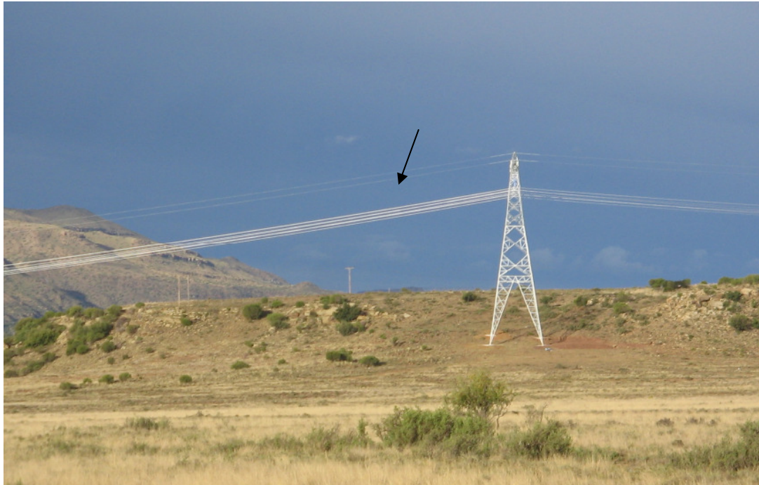
Figure 16. A 400 kV line, with all conductor wires in the same horizontal plane. This picture also demonstrates the almost invisible thin earth wire (black arrow) in top (Photo: EWT-WEP).
