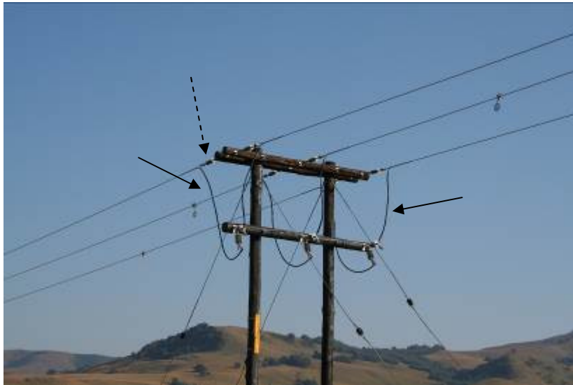
Figure 8. A safe strain pole structure, with insulated jumper wires (black arrows) and sufficiently long insulators (broken arrow) (Photo: EWT-WEP).
