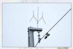
The wishbone prevents birds from landing above the wires
