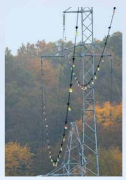
The bird flight diverters improving visibility of highvoltage electricity transmission lines in Kaunas near hydroelectric power station
