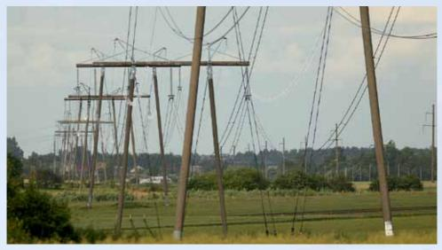
Visibility of wires improved with the help of white coils
